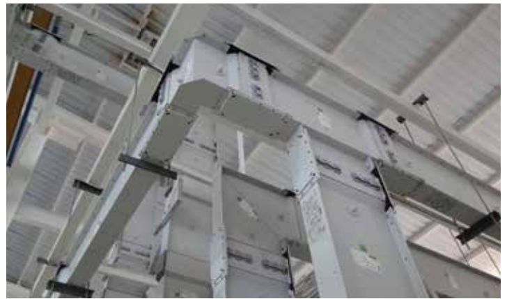
Example of Legrand busbar system
